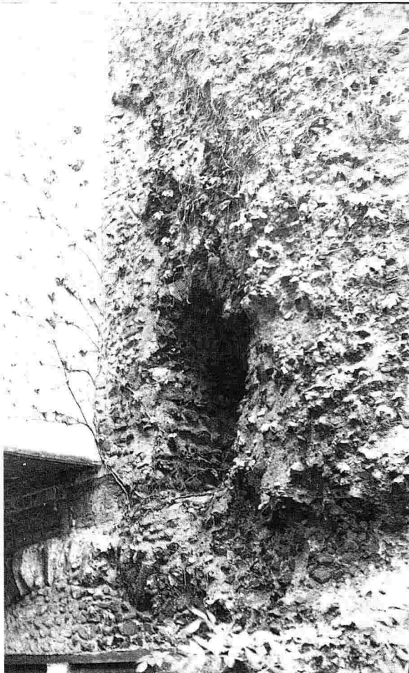
FIG. 37 – South face of north wall of north chapel block, with the short opening through the wall above the arch (lower left) of the former corridor leading to the (destroyed) northern octagon [Fig. 24A, x] ( photo: author ).
