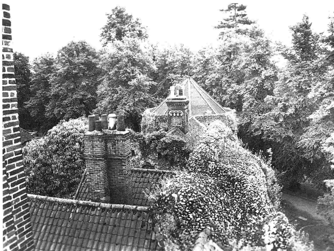
FIG. 34 – View over house roof tops to western half of south end wall of transept and south octagon ( photo: author ).
