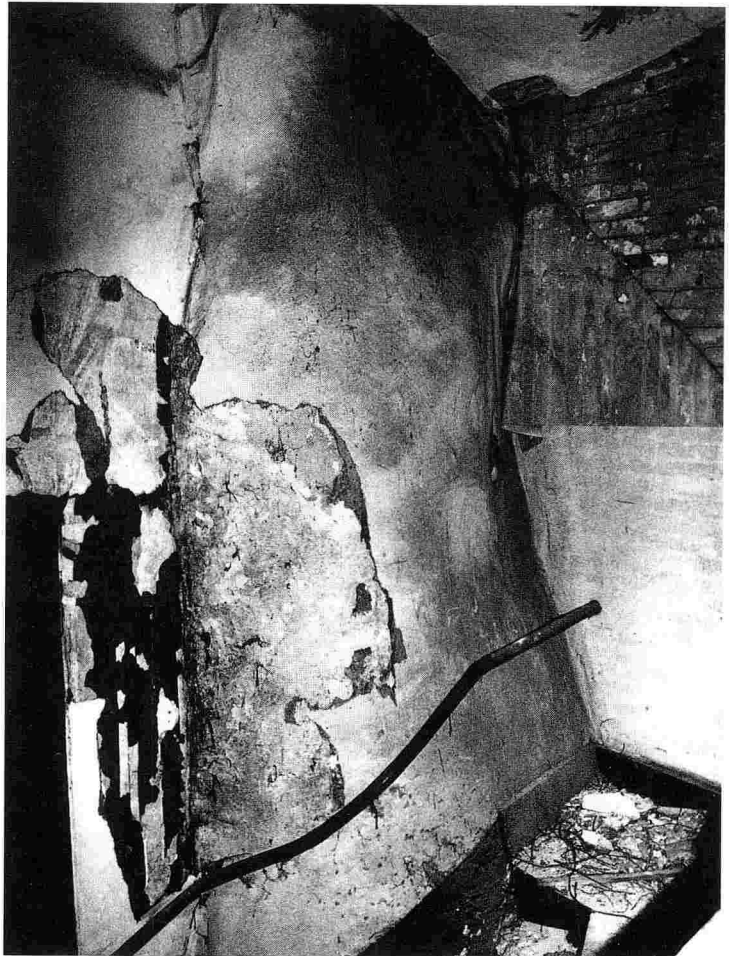
FIG. 31 – Mass of north-west respond of west tower hidden under plastered lathing in staircase of house No. 1 [ k in Figs. 24B and 24C] (photo: author).
