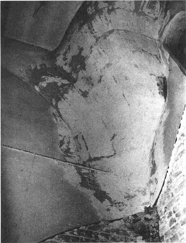
FIG. 35 – Springing of 12th-century groin vault inside house No. 3 at north-east corner [Fig. 24B, between t' and u'] ( photo: author ).
